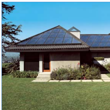
Sharp's triangular modules with black frames, trim strips, and backing sheets allow for the seamless integration of the system into the home's design.
